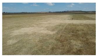
The main N/S runway with top soil filling holes & depressions mainly along the western side. Some soaking rain would be nice now to consolidate the fill.
