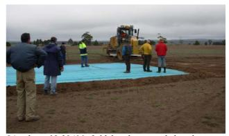
It's about 10:30AM, field has been graded and matting laid out ready for the edges to be buried. Craig is backfilling the western end with the grader blade under the scrutiny of many watchful eyes.
