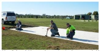
Mat, Rob and Max are hammering in the pegs to hold down the sides if the matting. (About one per metre)
