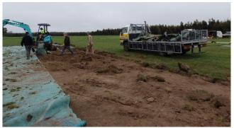
The Kobelco with Martin at the controls made light work of a rather daunting task. When the matting was laid the grader went along the edge of the strip with the blade on an angle to dig a trench. The edge of the matting was laid in the trench then the grader back filled locking it into place. After several years of grass growing through it, it was just impossible to pull out by hand.
