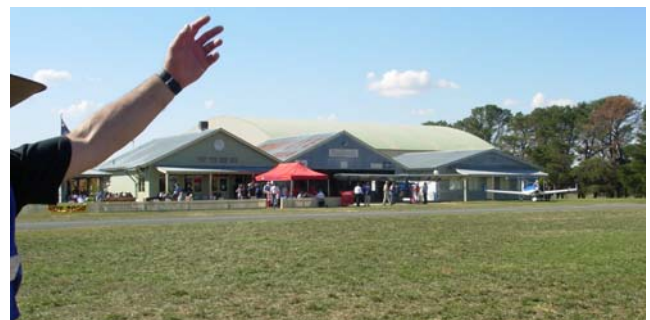
The restored Bowlye Flying Club facilities. Sorry for the arm($#@%) – it's the only photo I had.
