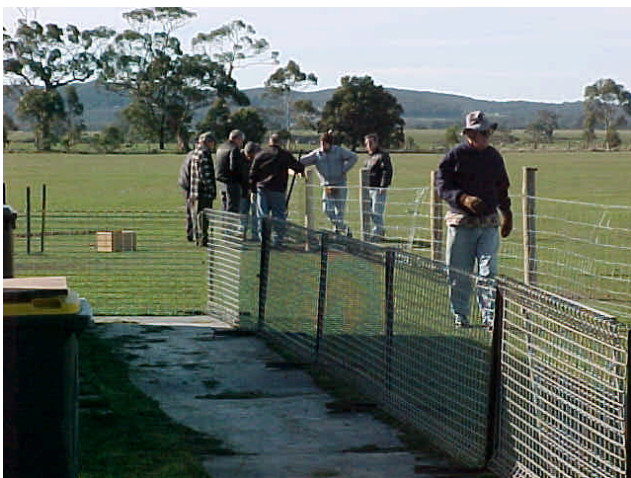
The old temporary fence has now been removed.
