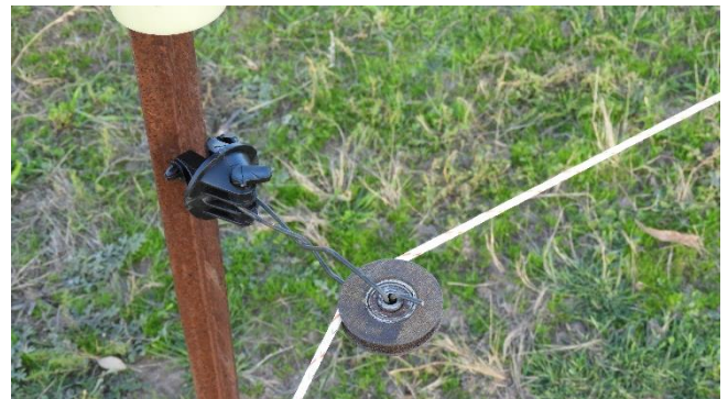
One of seven cables fitted to the corner posts – four down the southern end, two at the north/east corner and one where it runs across at 90 degrees to the power unit.
