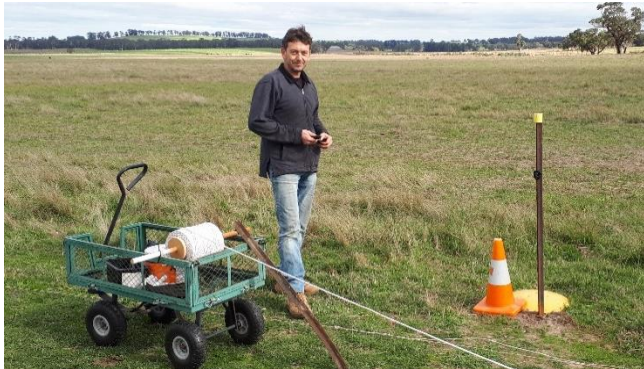
After picking up the cable from Hewitt & Whitty I found a length of 1" dowel in the garage and cut out two big washers from MDF scrap thinking we'd be hanging onto it while rolling out. Al suggested tying it to the trolley which worked a treat. Al is bending the wire to attach the pulley.
