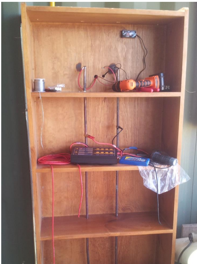
A charger connected to the charging bus using the clips the charger comes with
