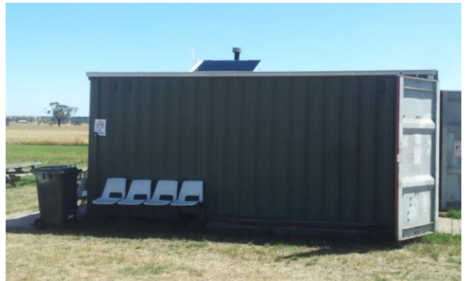
The solar panel was mounted on the roof of the container pointing in a generally northerly direction.
