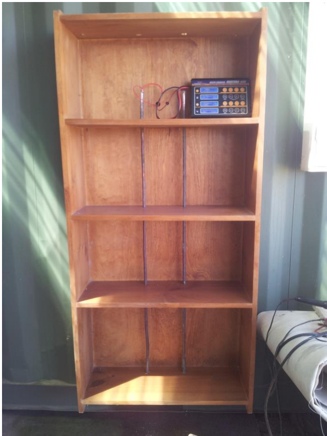
Charging station built into a disused bookcase cabinet which has been mounted to the wall of the container which is under the covered in area.
