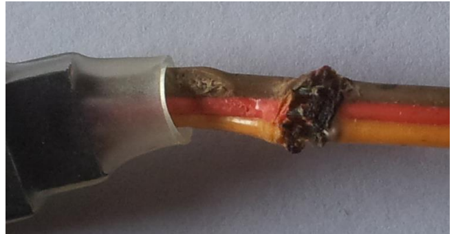
A close up shot of the melted battery lead caused by the lead rubbing through the insulation inside the fuselage. Must have rubbed on something metallic like the throttle pushrod.
