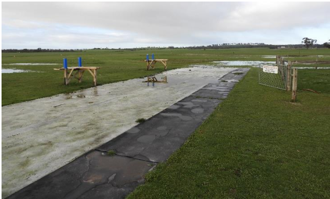
There's a depression along the pits that we reckon will take a couple of cubic metres of granite sand to fill before the replacement matting is laid. (Near photo centre)
