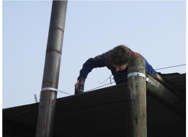
Alan volunteered to go up on the veranda roof and resecure the flue.
