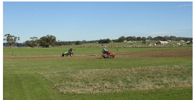
Murri and Peter W. smoothing out the runway extension with the mowers. Photo looking south and taken on Sunday 9 th June.
